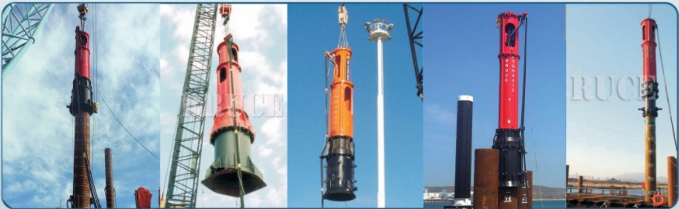
Hammers working with crane suspended type.
